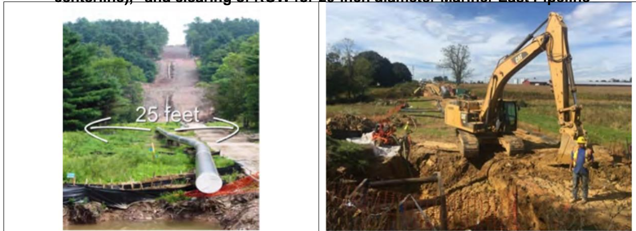
Figures 2a and 2b. typical Pennsylvania 15-meter pipeline ROW (25 feet on either side of centerline), 8 and clearing of ROW for 20-inch diameter Mariner East Pipeline 9
